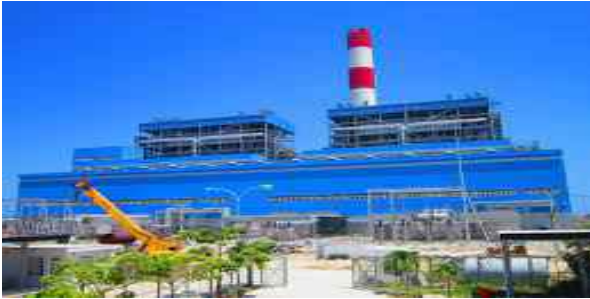
Vinh Tan thermal power plant Contractor: Posco E&C - Korea
