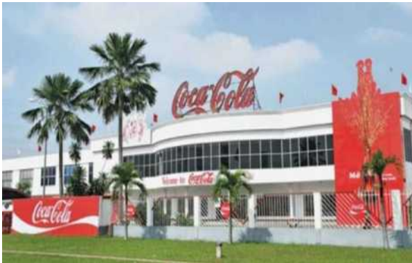
Coca-Cola Hà Nội plant Contractor : Probuild
