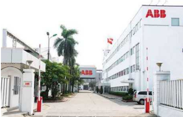
ABB Việt Nam plant Contractor : Unicons - Vietnam
