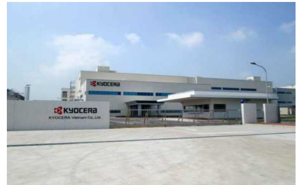
Kyocera plant Contractor : Kinden - Japan
