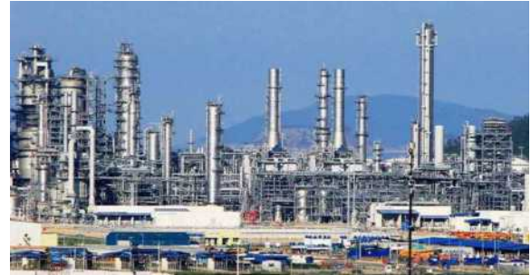
Nghien Son, Long Son oil refinery plants Contractor: Temsco - Korea Contractor: Deasun - Viet Nam
