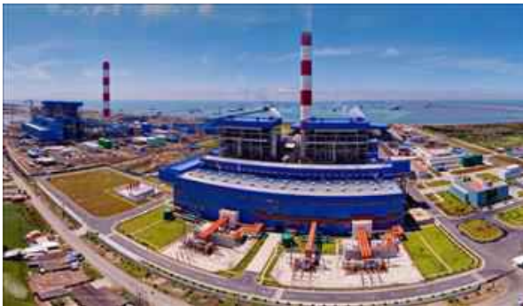
Thai Binh thermal power plant Contractor : Sigma - Vietnam
